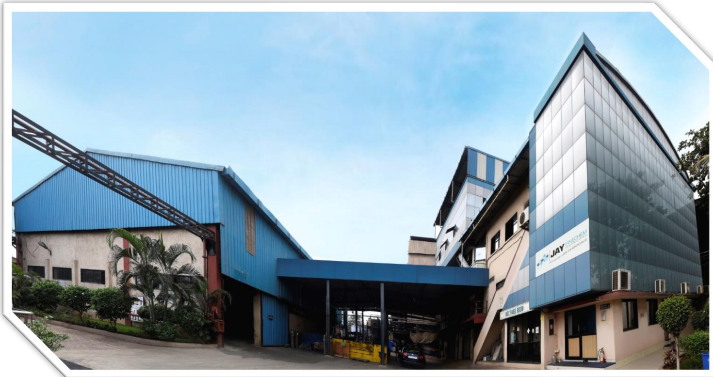
Jay Finechem Plant
